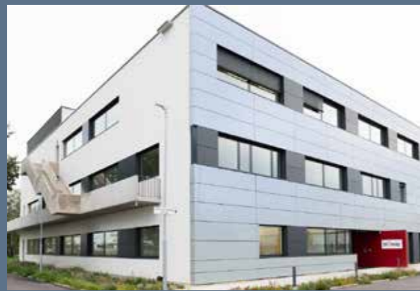
VTU planned and built a state-of-the-art biotech facility at the Biomay site in Vienna.
