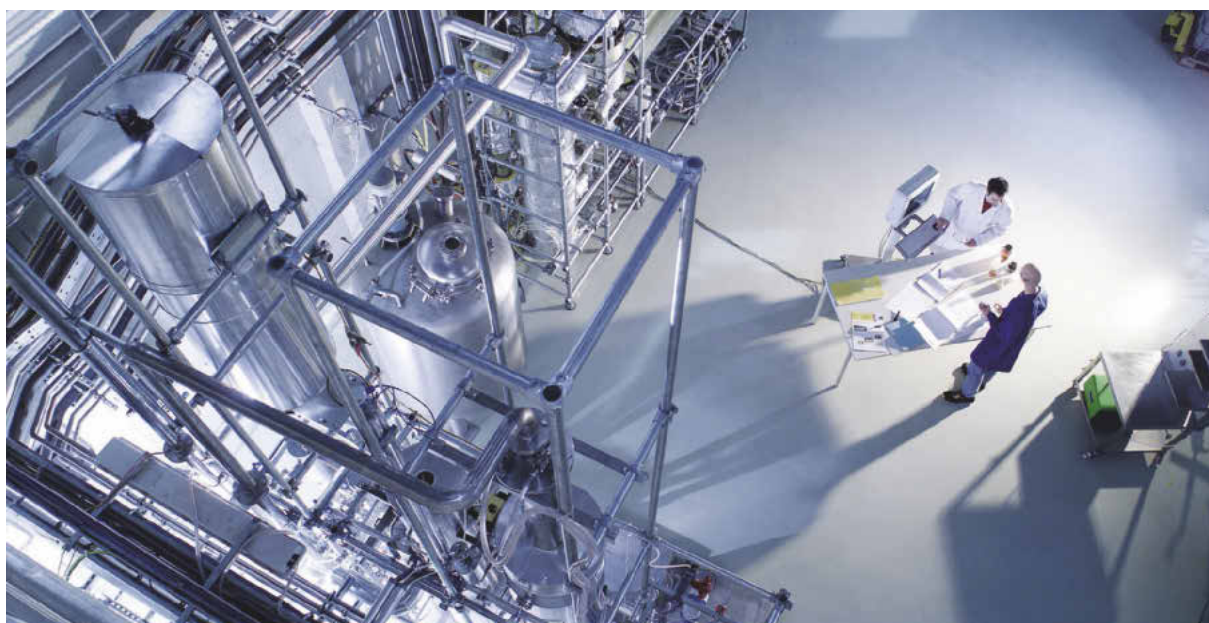
Blick in das Technikum von VTU Engineering in Graz
